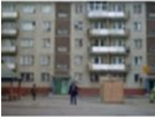
a block of flats
